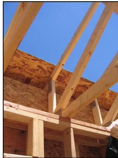
Fig. 4: Raised heel trusses
